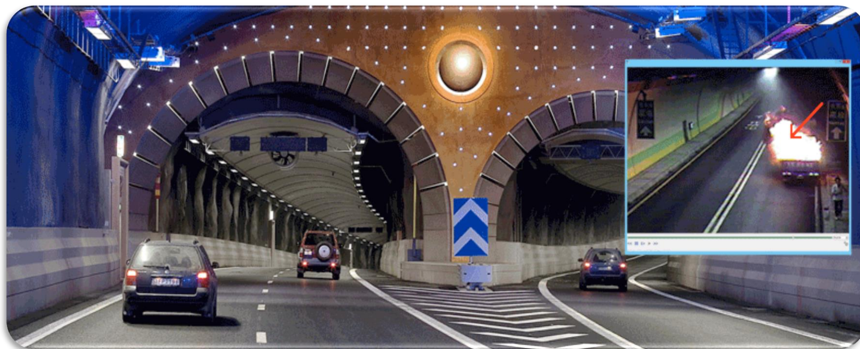
Incident detection application in tunnel.
